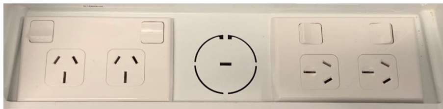
Figure 6. Power points with different orientations
