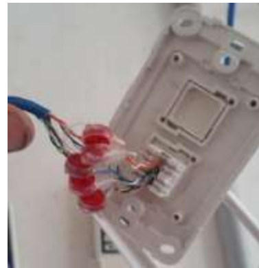
Figure 5. Example of Substandard Cat6 Cable Crimping & Punch Down
