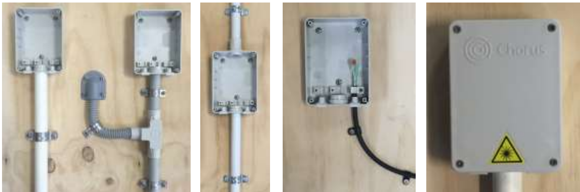
Figure 2. Example of ETP Mounted on Walls
