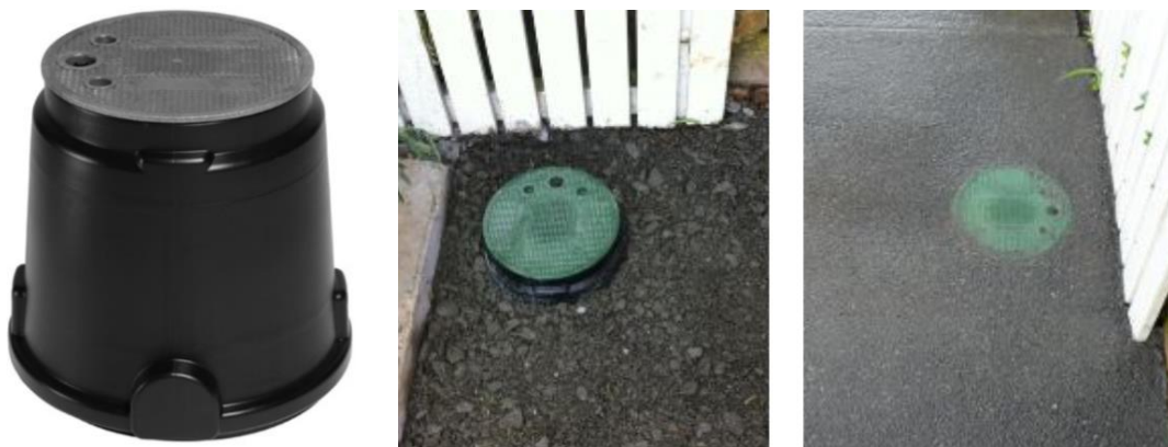
Figure 1. Channell Handhole at the Premises Boundary
